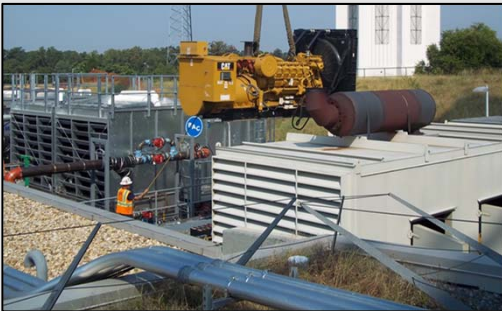
UPS and backup generators installed at Suitland, MD
